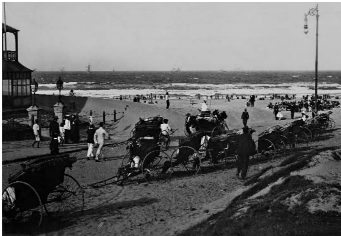
Durban beach. Rickshaw are the only means of transport. Sailing ships and steamers are anchored offshore waiting for a berth
